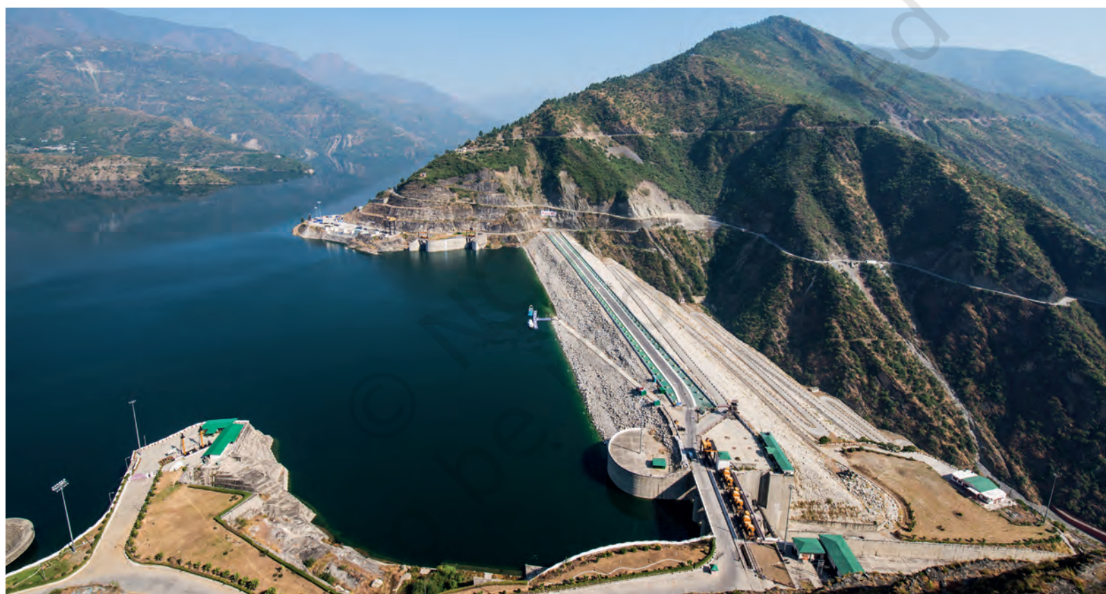
Figure 6.1: Tehri dam in Uttarakhand
