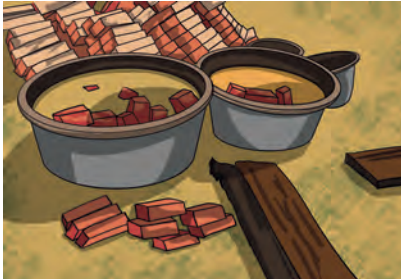
Figure 6.14: Bricks are soaked in water before use
