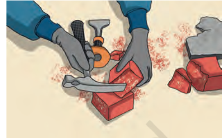
Figure 6.16: Cutting the brick using chisel and hammer
