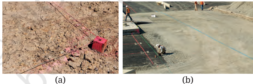
Figure 6.13: (a) Using reference lines for marking site of construction, and (b) marking lines for construction
