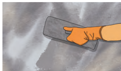
Figure 6.19: Applying plaster on the wall
